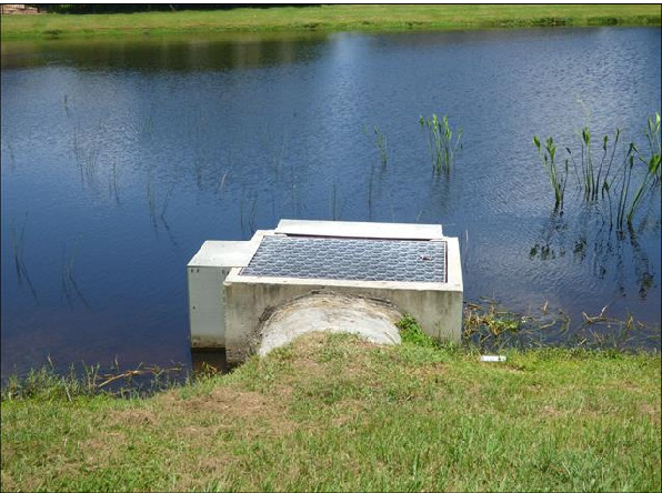
Stormwater Drainage Control Structure
